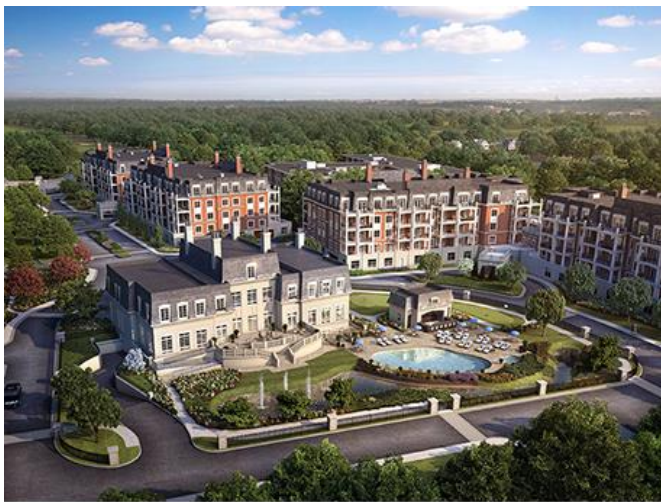
The Ritz-Carlton Residences, Long Island, North Hills are located 20 miles east of Midtown Manhattan on Long Island's North Shore.
