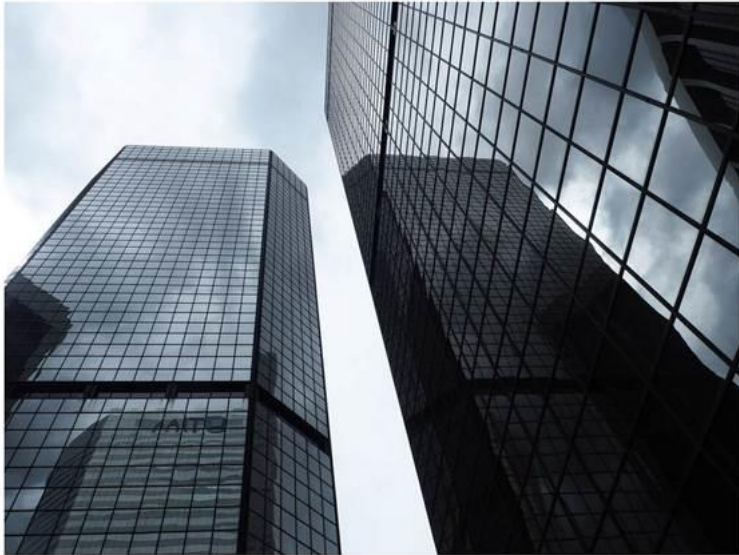
Lenders have seized office buildings such as the former Denver Energy Center, seen here in April 2022. Photographer: Thomas Gounley/BusinessDen
